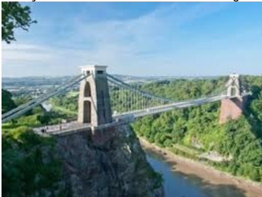
Clifton Suspension Bridge – I K Brunel's famous landmark spans the beautiful Avon Gorge
